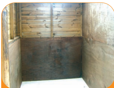
6' Store Room internal
